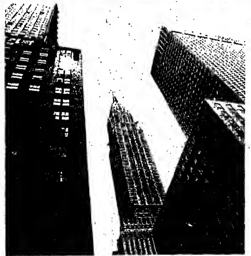
The Empire State Building
